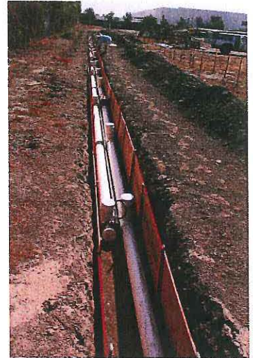
Horizontal Extensometer Construction
